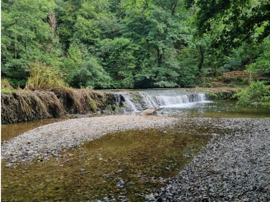
Figure 1. Photograph of weir (Case Study One).
