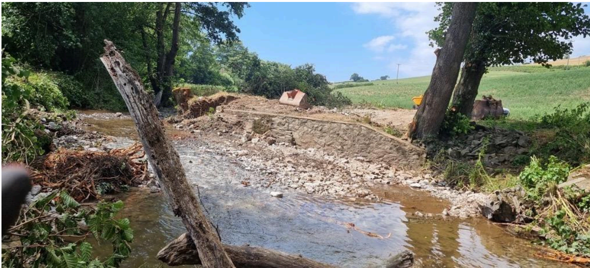
Figure 5. Chipley weir directly after removal.
