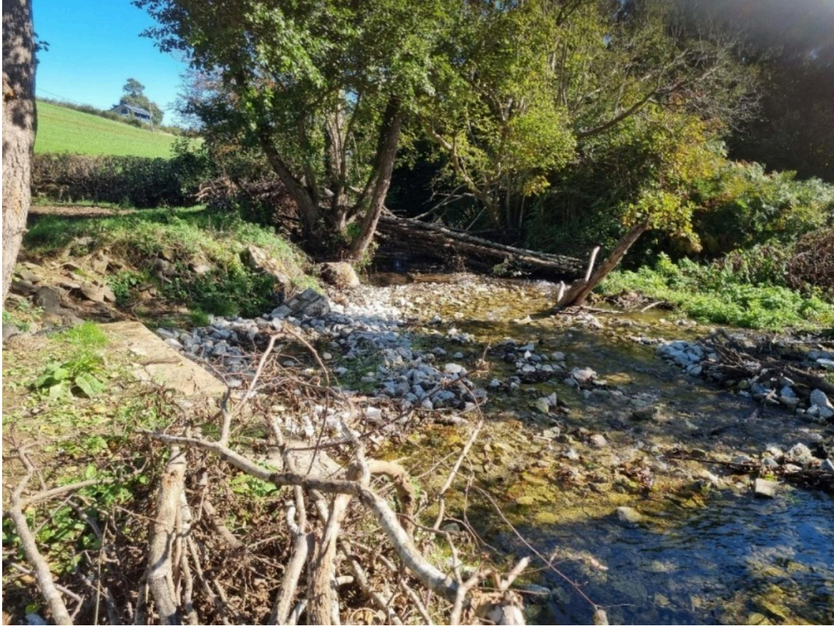
Figure 6. Chipley weir downstream view around 1 month post removal.
